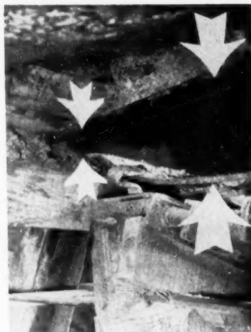
This eight-inch steel cap, used above one of the grizzlies feeding a conveyor in the Miami Copper Company's mine, has been compressed to a third of its former web thickness by the nearly irresistible weight.
